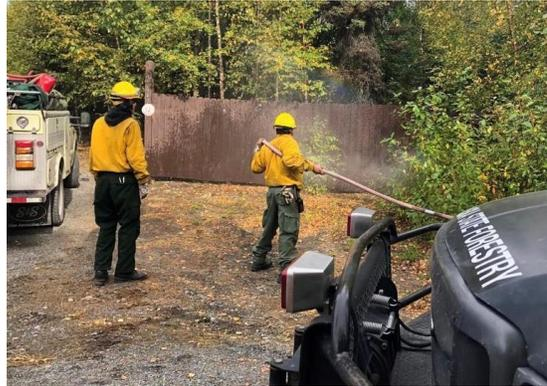
*Firefighters assigned to Cooper Landing train on sprinklers installed for exterior structure fire protection.*
